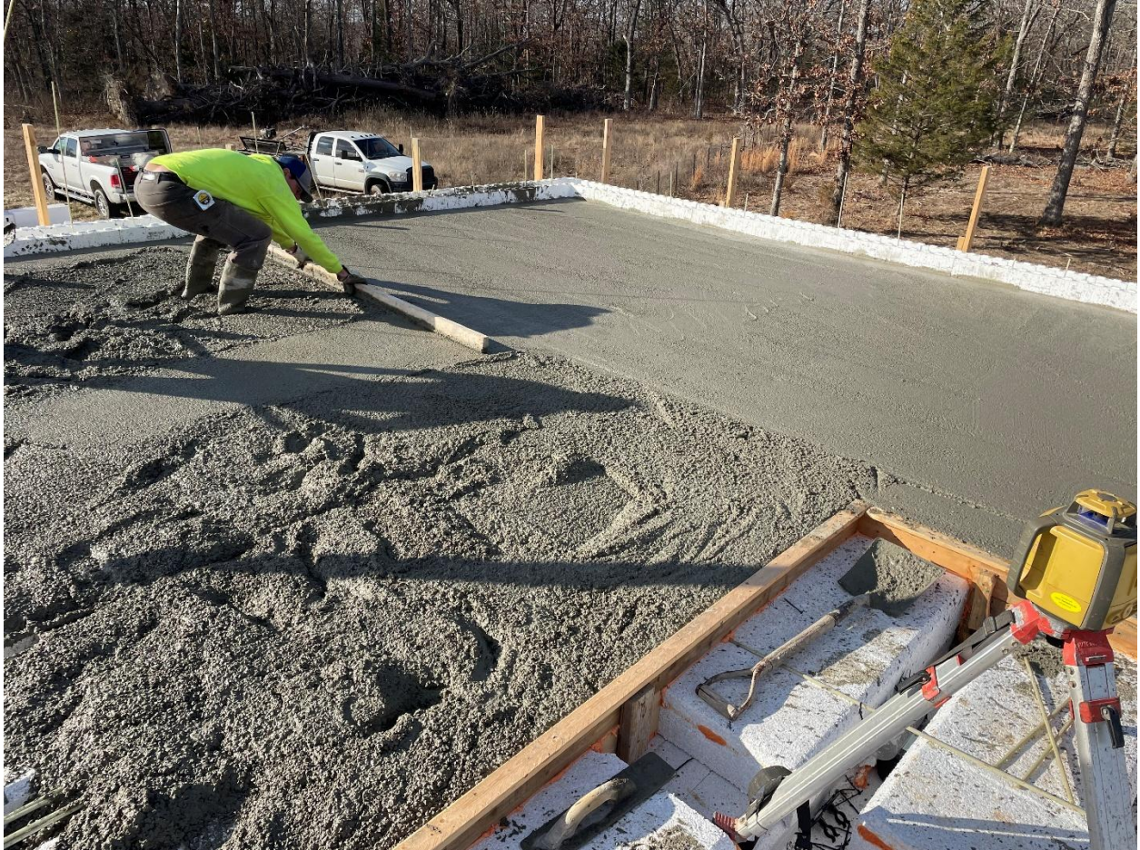
Figure 7 Image of second story slab in progress
