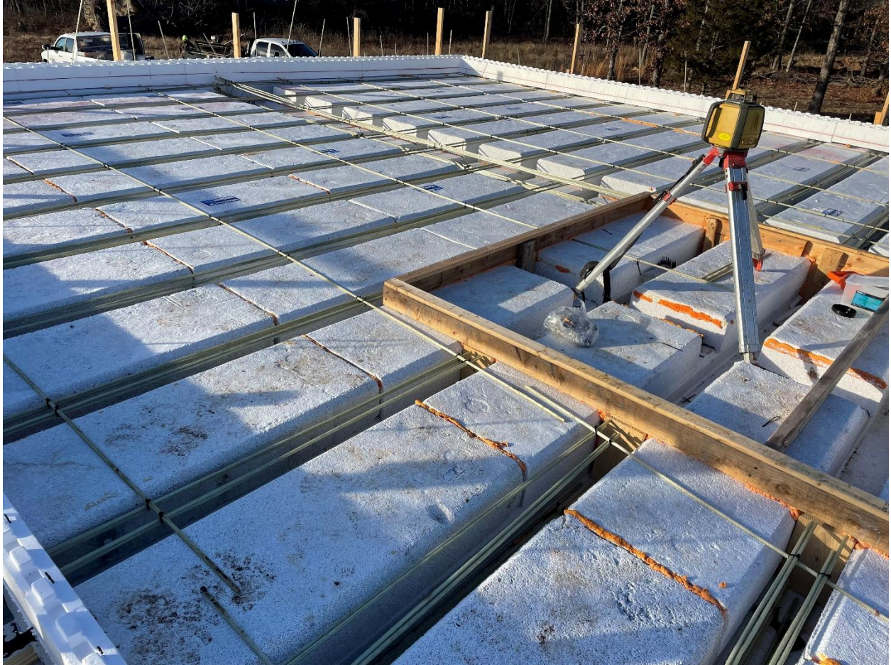
Figure 13 Image showing second story preparation prior to slab pour
