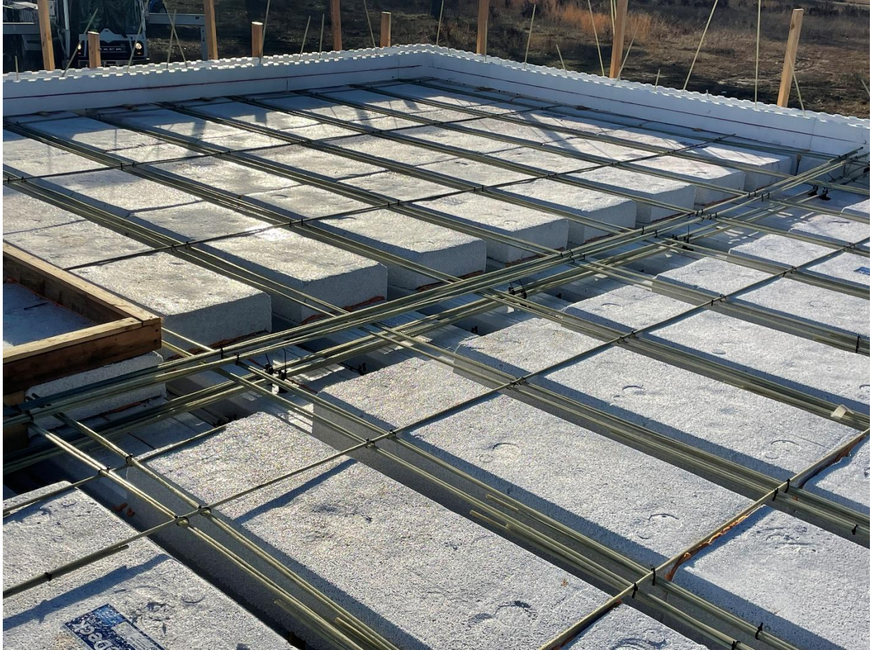
Figure 10 Image showing excessive tied rebar in place prior to pour
