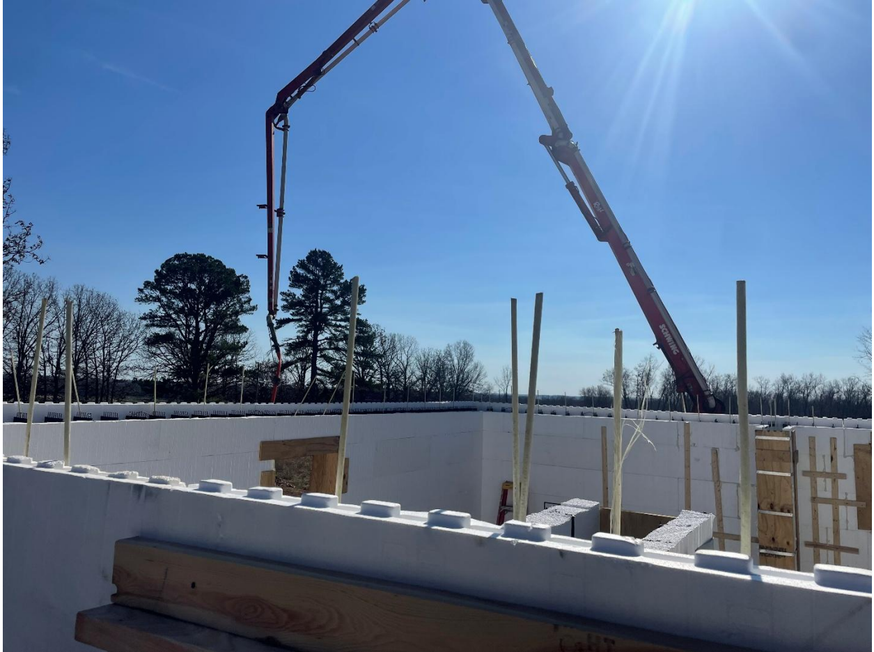
Figure 8 image showing vertical rebar
