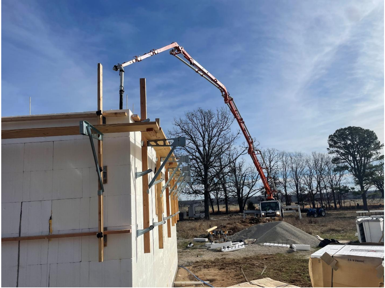
Figure 5 Image of pump truck preparing for concrete
