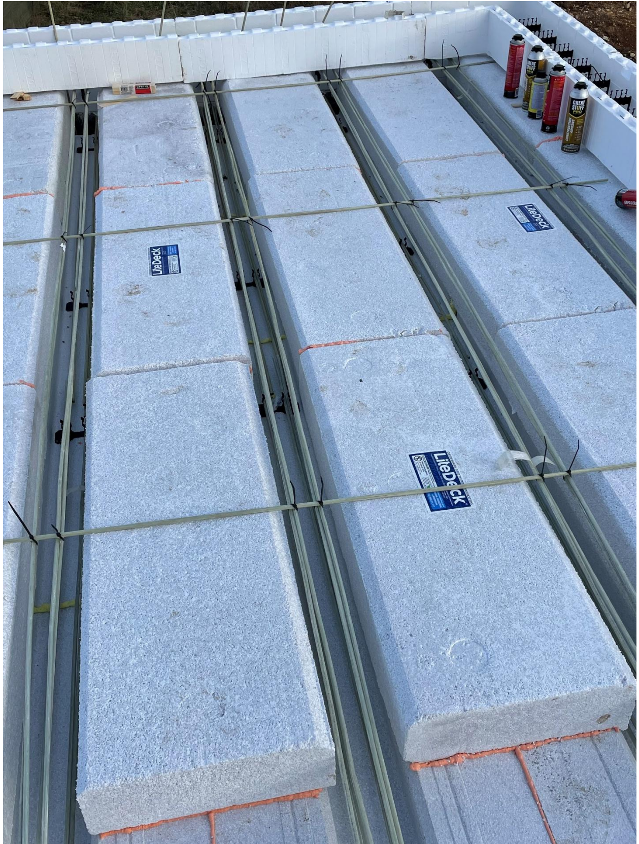
Figure 14 Image showing second story prep prior to slab pour
