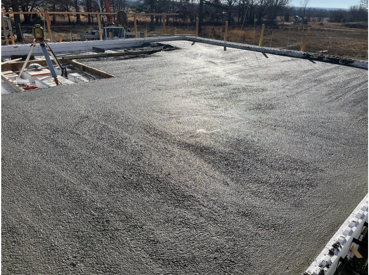
Figure 6 Image of second story concrete slab prior to finishing
