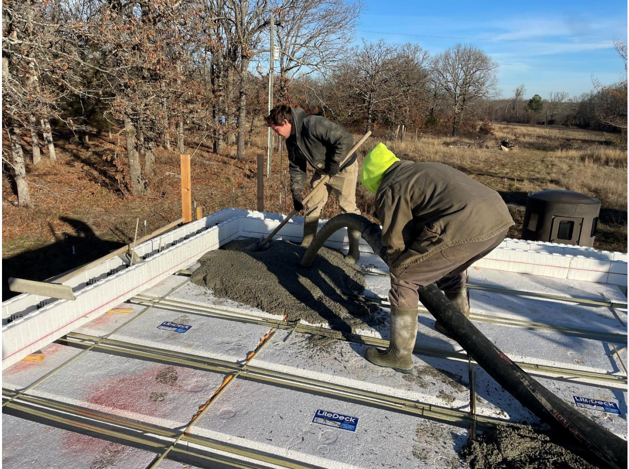
Figure 9 Image showing second story slab in progress
