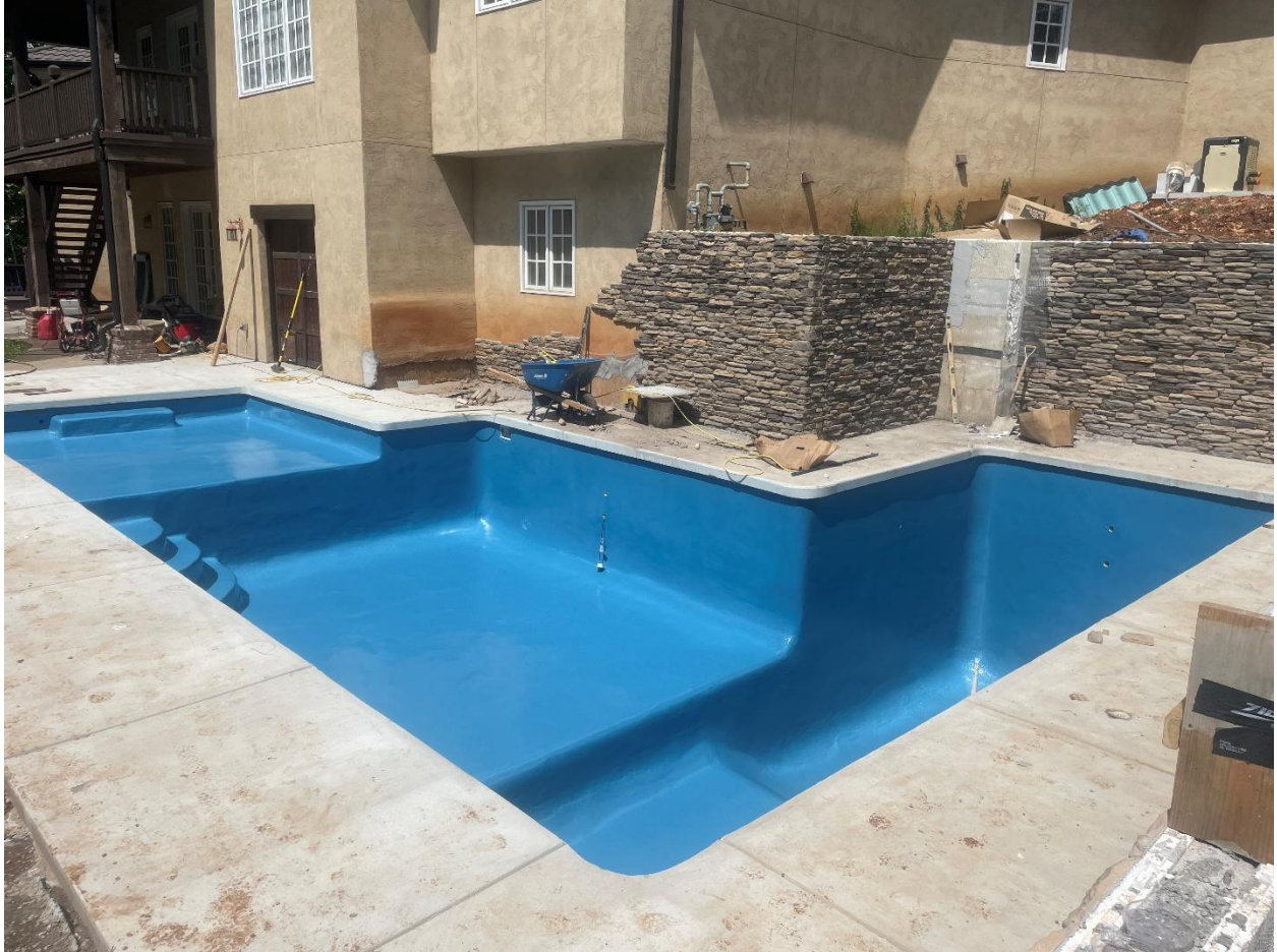
Figure 3 Photo showing completed interior and nearing completion of retaining wall
