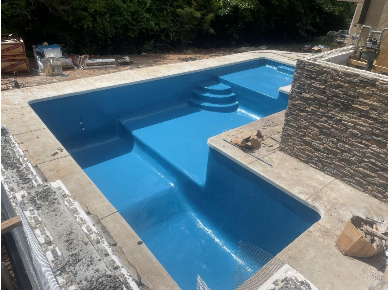
Figure 2 Picture of the pool as its nearing completion. One of the final two photos taken just prior to the unexpected confrontation with Emily Smith.
