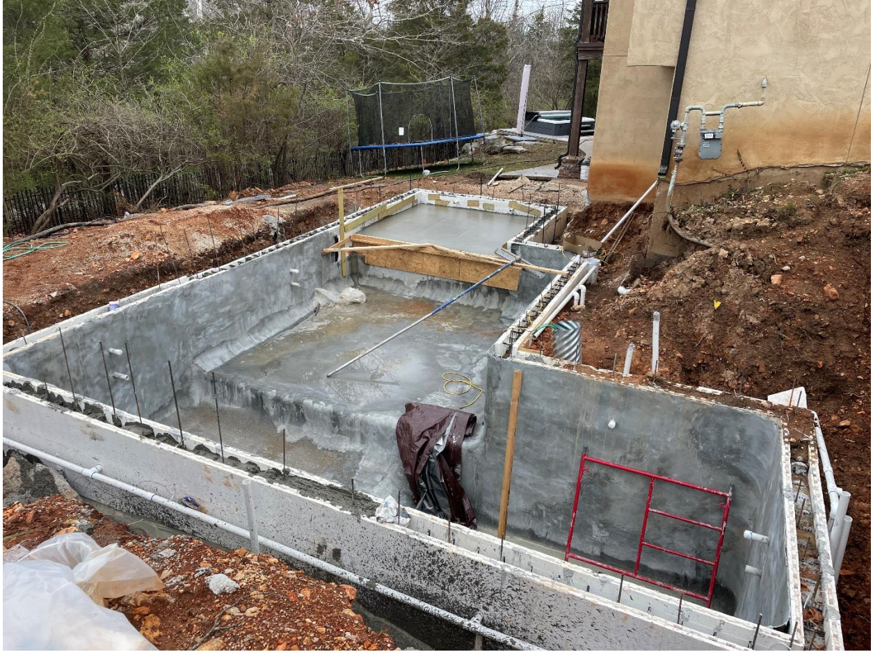
Figure 6 Photo showing interior Hard Shell Liner nearing completion
