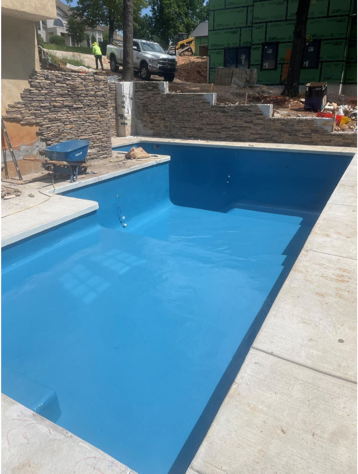
Figure 4 Photo showing completed interior and nearing completion of retaining wall
