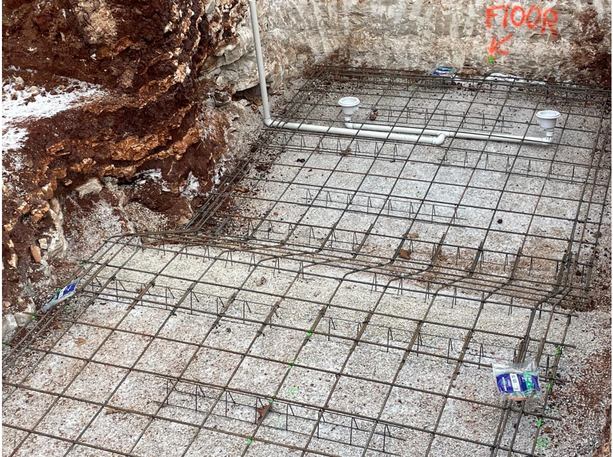
Figure 10 Photo showing #5 rebar 12" on center in deep end
