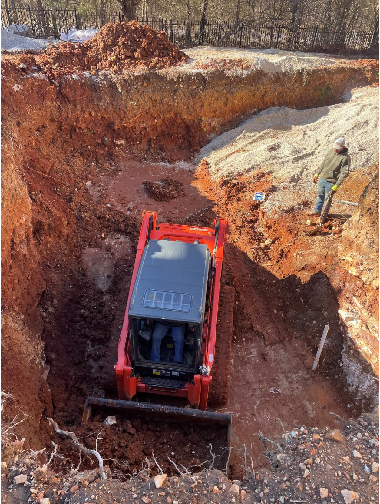
Figure 8 Photo showing excavation just prior to hitting solid granite shelf rock
