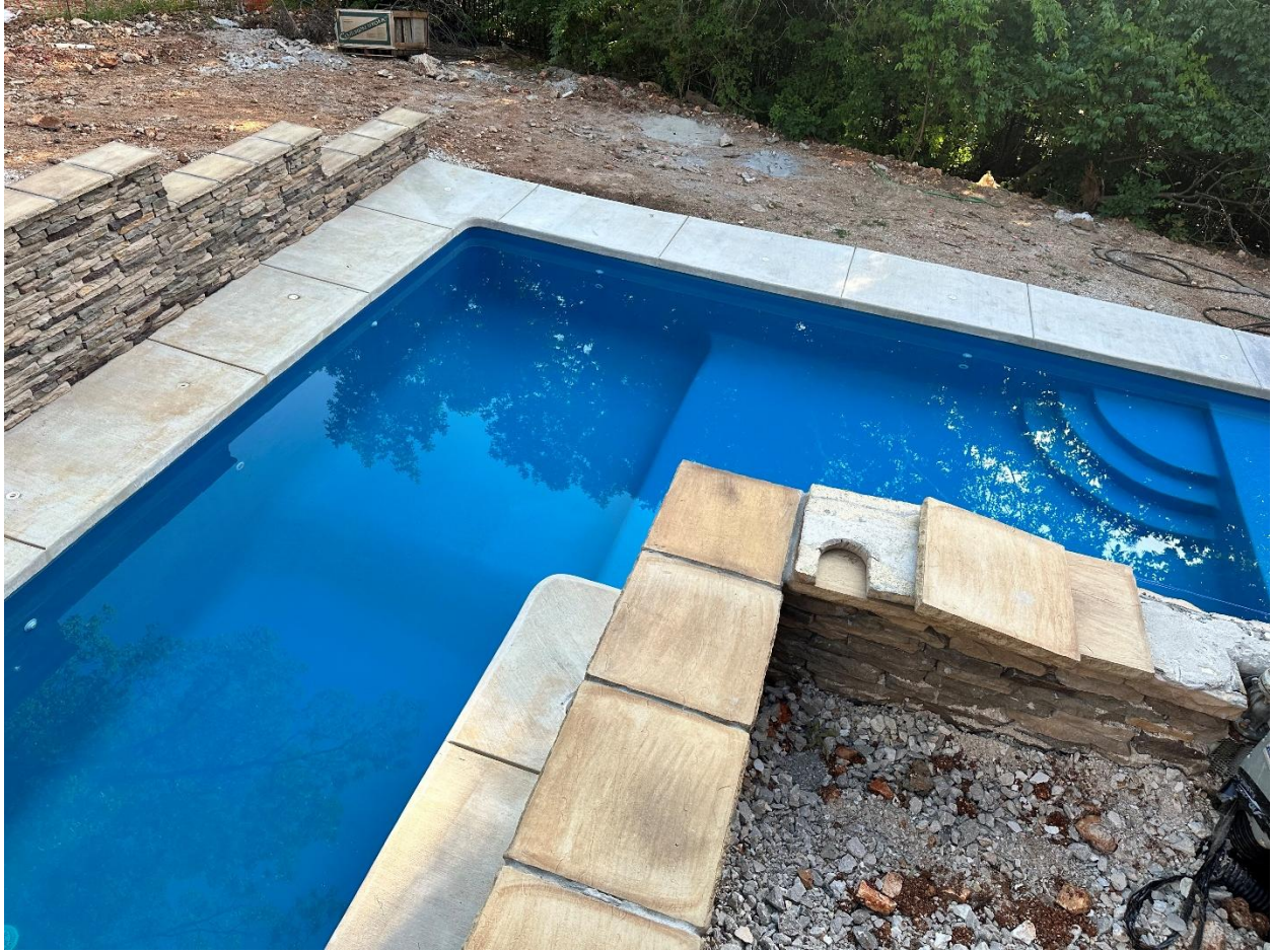
Figure 1 Picture of the pool as its nearing completion. One of the final two photos taken just prior to the unexpected confrontation with Emily Smith.
