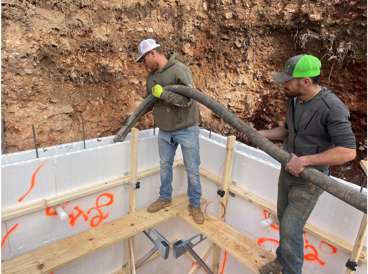
Figure 7 Photo showing workers pumping concrete into the wall forms
