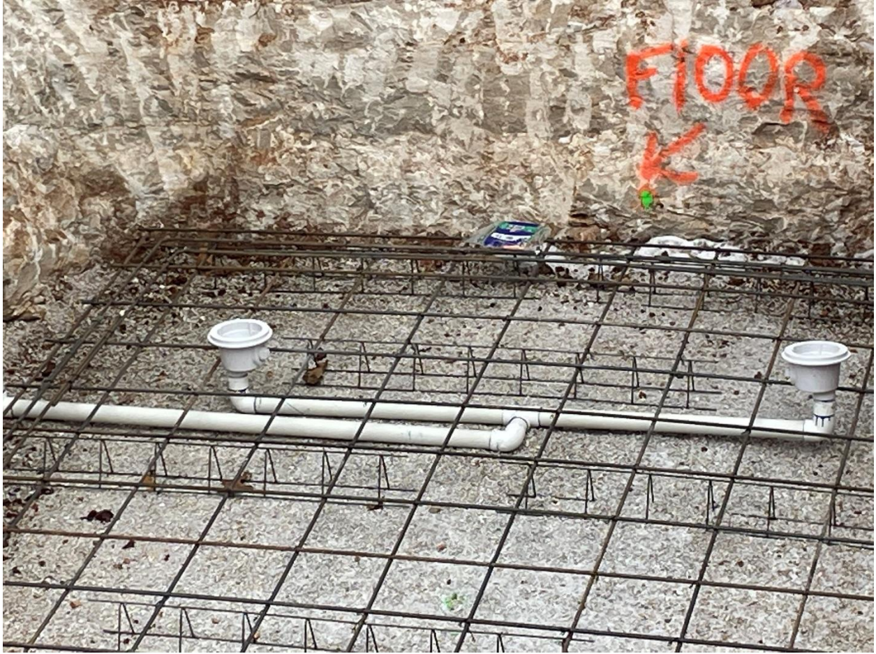
Figure 9 Photo showing drain pipes secured in place and exposed shelf rock
